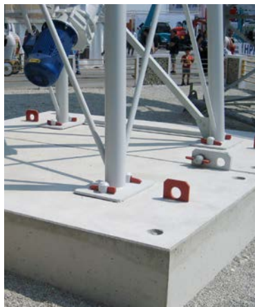
Mobilfundamente Mobile foundations
